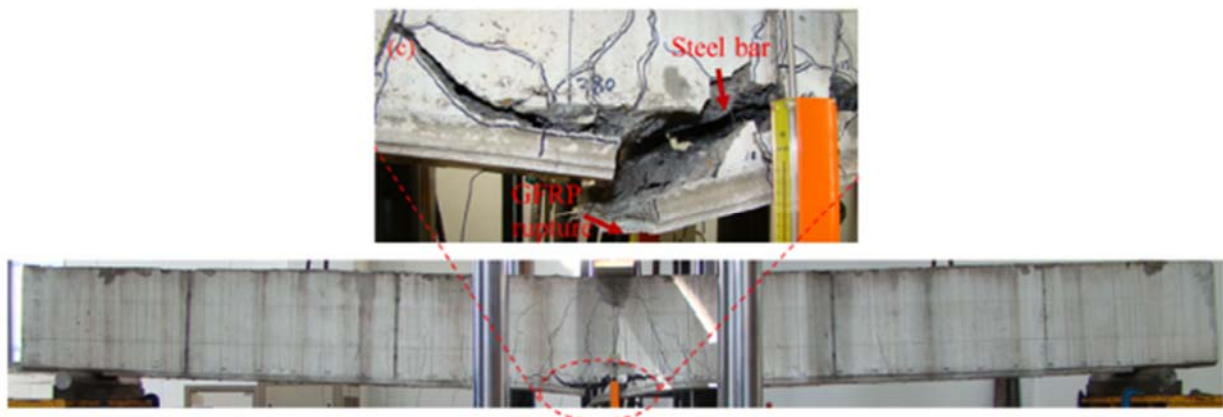
Figure. 15-year-old RC beam strengthened with FRP composites at failure
