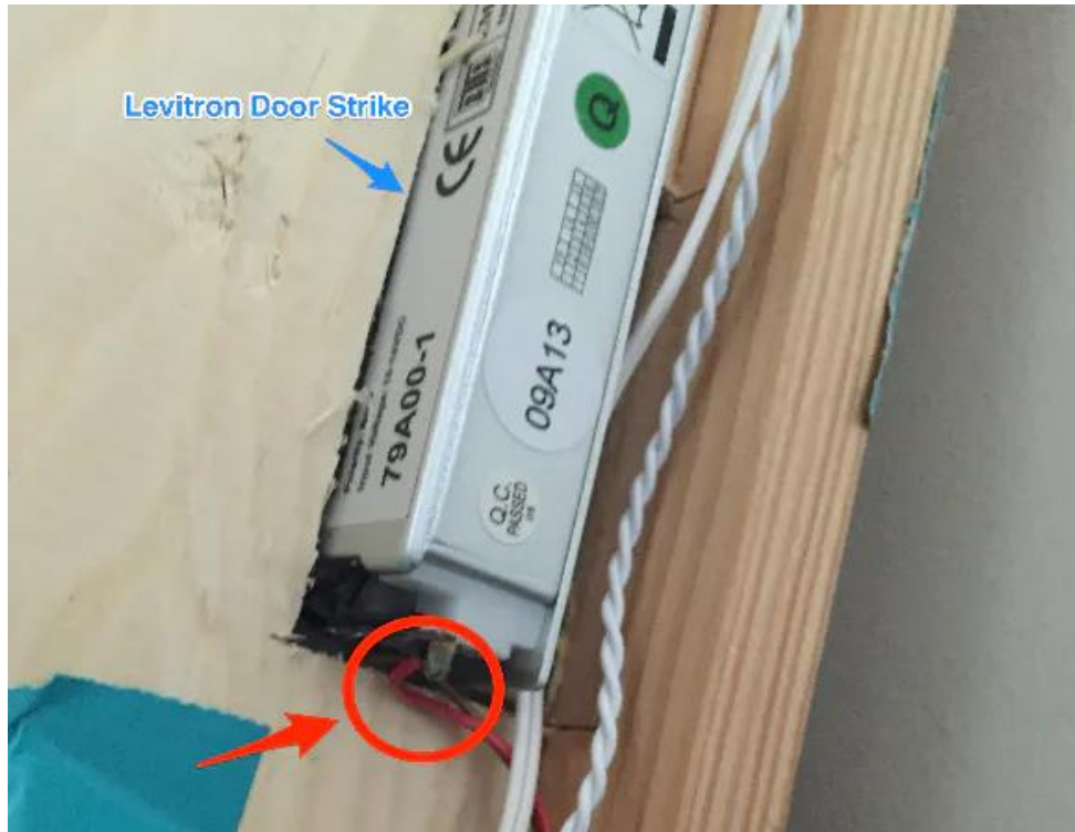
Figure 5- The picture shows the door strike and wire connection from the relay.
