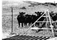
Cow grate at fence openings
